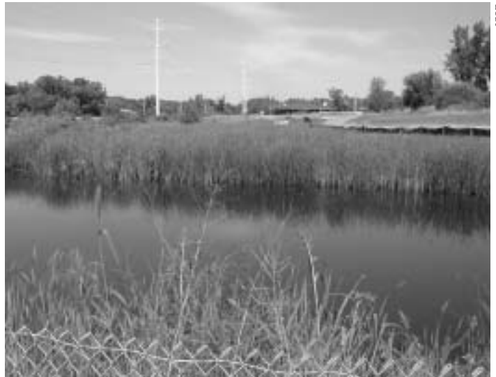
AFTER: By August 2003, the Bartlett Brook constructed wetland teems with vegetation that will help filter polluted stormwater runoff.
